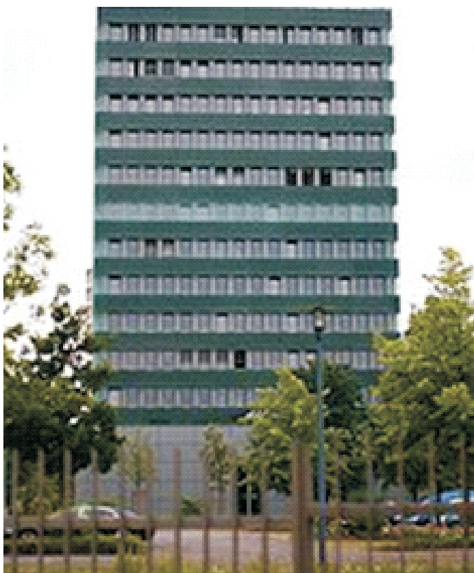
German Federal Ministry of Health Office Building, Bonn
