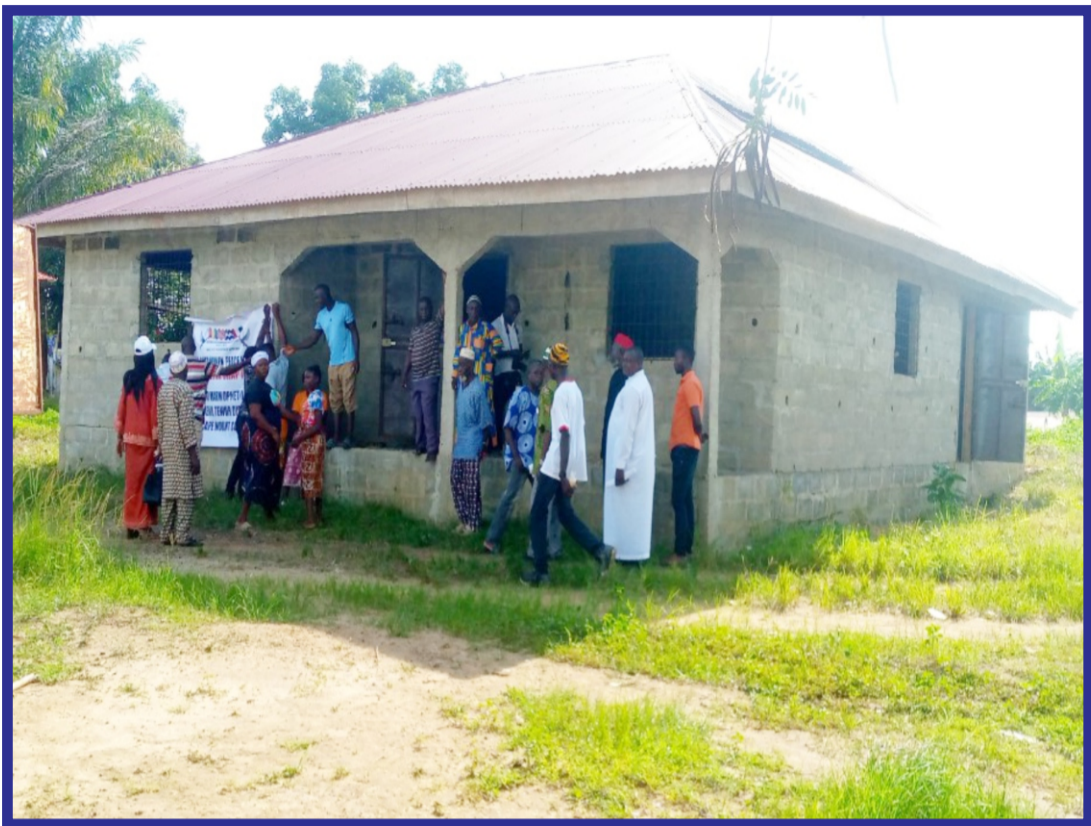
Newly constructed MARWOPNET station
