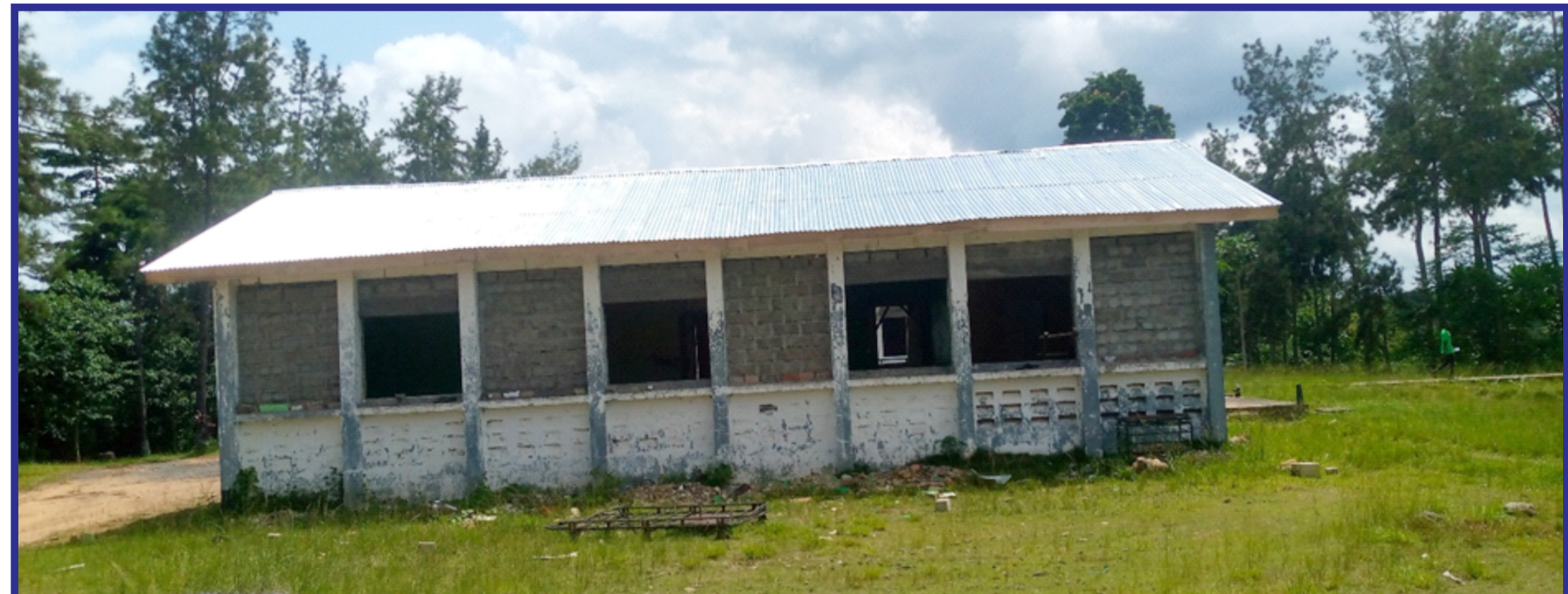
Constructed FTI building in Bomi County
