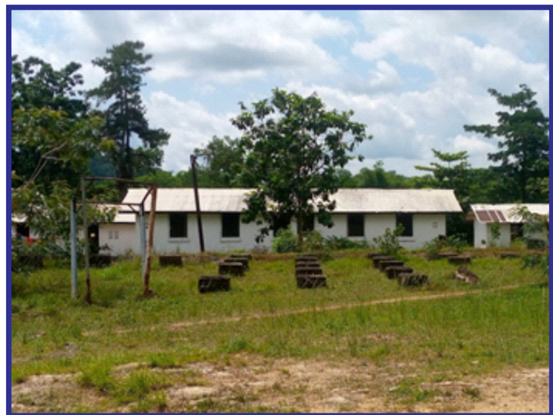
Some structures at FTI in Bomi County
