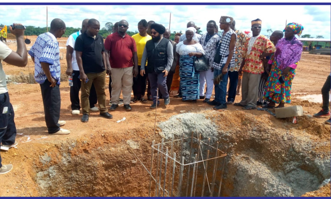
Mr. Jeety and elders at the construction site
