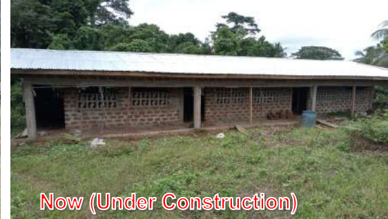
Under Construction, Nimiah Elem. Sch. In Grand Kru
